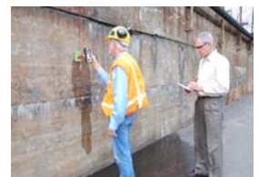
Half-cell Corrosion Survey
